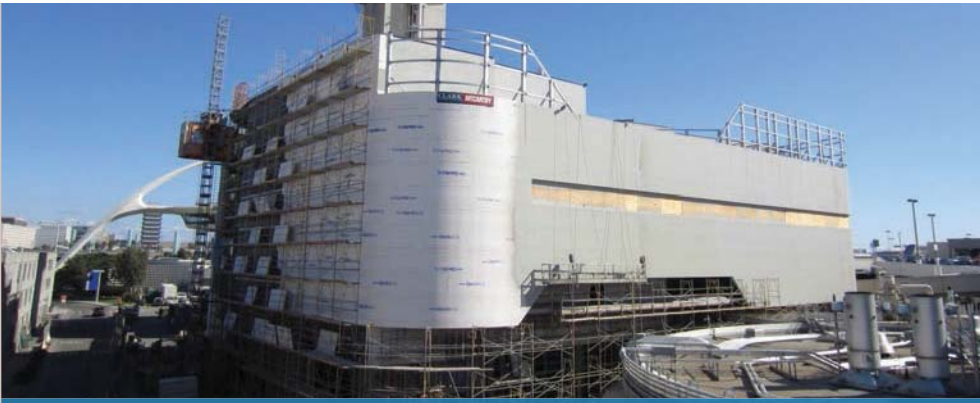
Central Utility Plant Replacement at LAX
