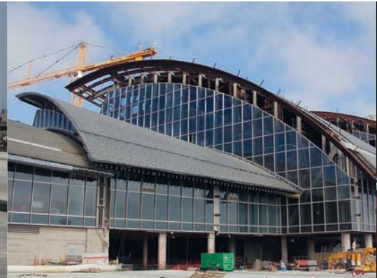
Bradley West under Construction (LA-Next Photo)
