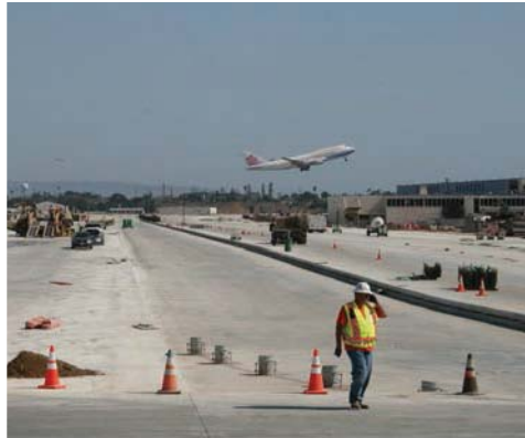
Construction on Taxiway S
